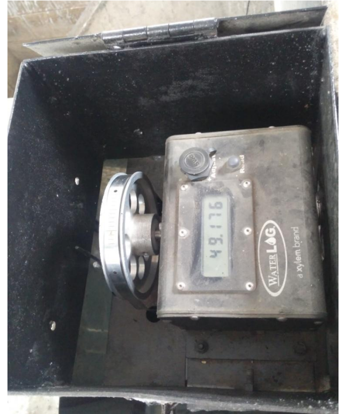
Shaft Encoder Type Water Level Sensor at Bhakhra Nangal Dam
