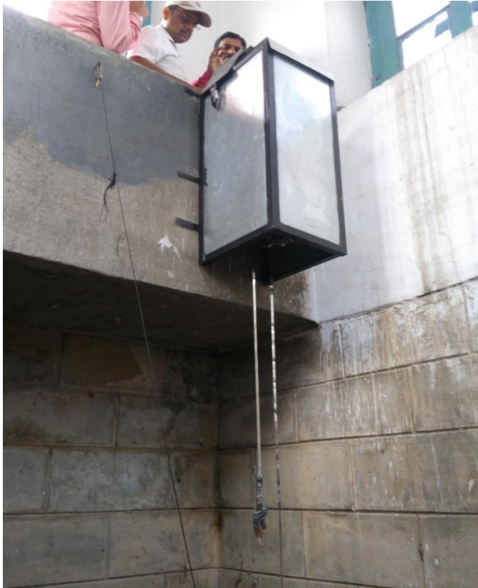
Shaft Encoder Type Water Level Sensor at Bhakhra Nangal Dam
